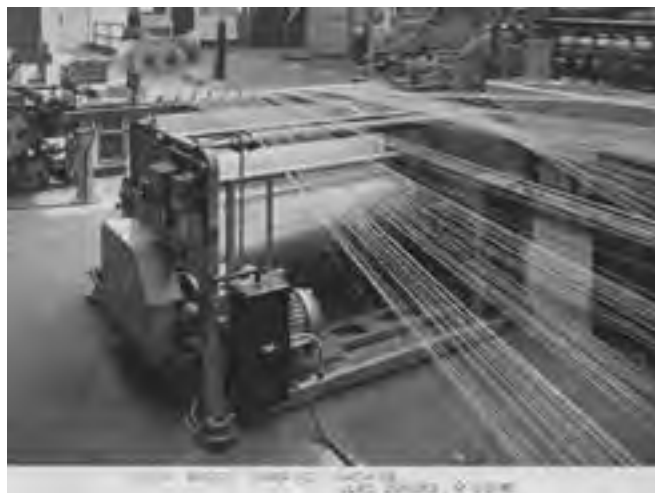
Urquhart Lindsay & Robertson Orchar, Ltd High Speed Warping Machine, Dundee Heritage Trust
