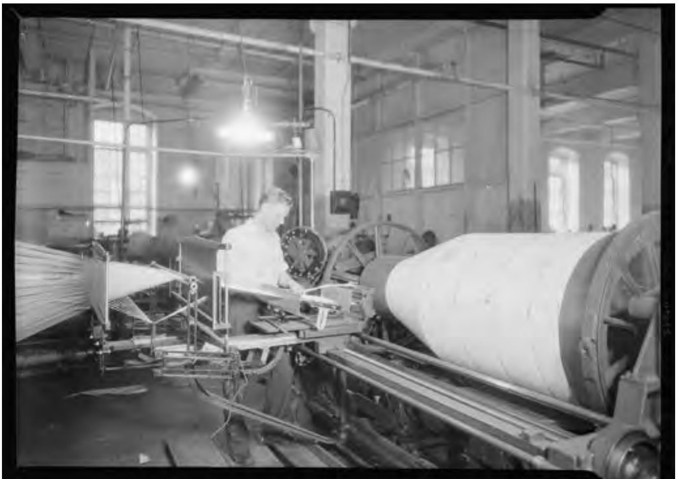
Jackson Winding and Warping Company, High speed warper, Paterson, New Jersey, 1937, Federal Works Agency
